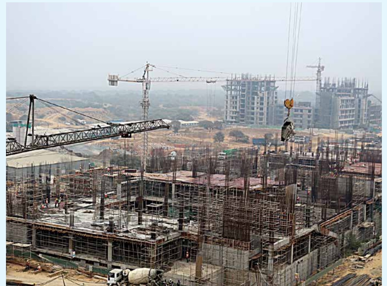
A view of the on-going construction of the campus buildings
