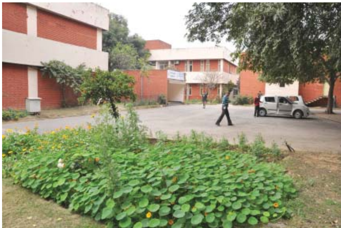
SAU building in JNU Campus
